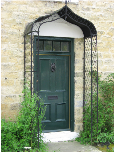
A beautiful example of a solid panelled door with fanlight over and an unusual lattice ogee topped porch
